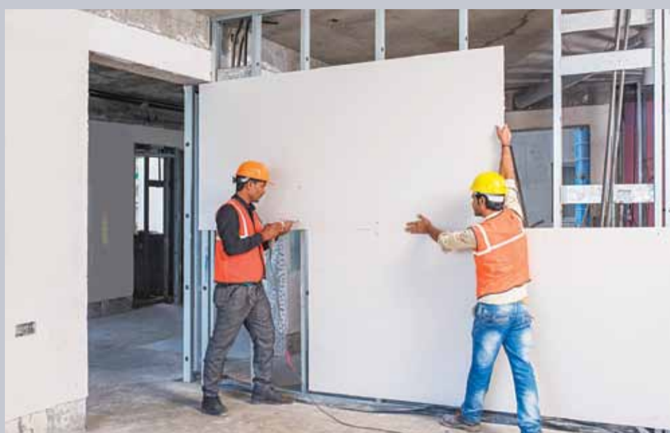
Path breaking "Dry Construction Technology" eliminates usage of concrete and brick; reduces water usage. Pre-fabricated bathrooms These are fitted directly into the apartments.
